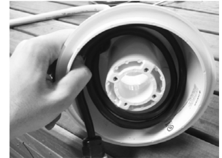
11. Pull the power cable through, leaving about 1m of cable to allow inspection of light above water surface.
