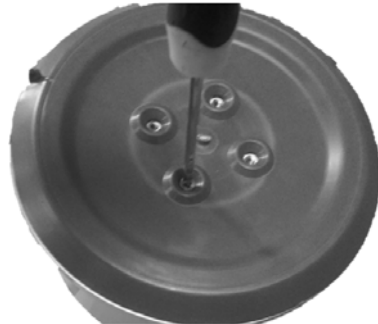
7. Attach the protection cover to the niche, line up the holes and use the included screws to secure in place.
